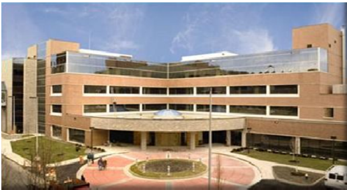
Figure 59: Existing Façade-View from Entrance
